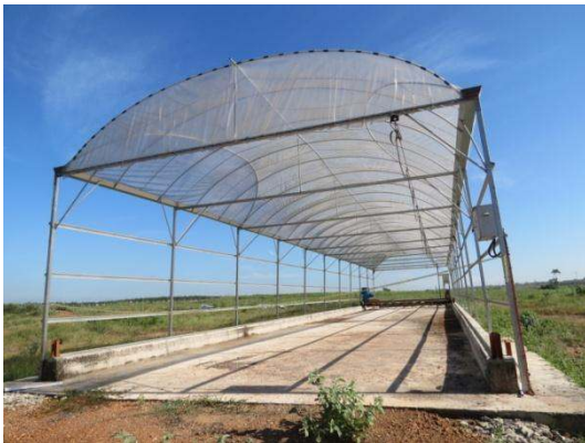
Gambar 5.1 Dryer - Cassava (Bahagian Dinding Rosak Ditiup Angin)
